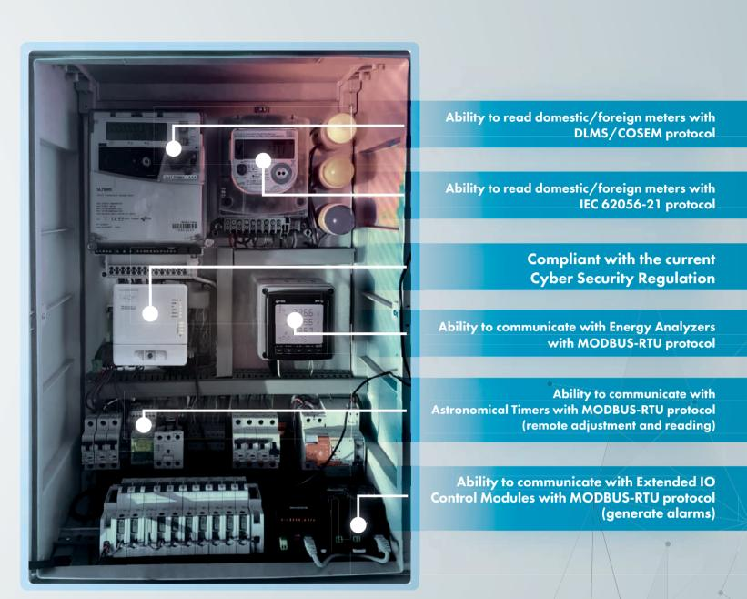
Thanks to the RS485 communication interface with improved ±35KV impulse resistance, sMOD-X can communicate with all the devices shown in the panel above over the same line (single RS485 line).
